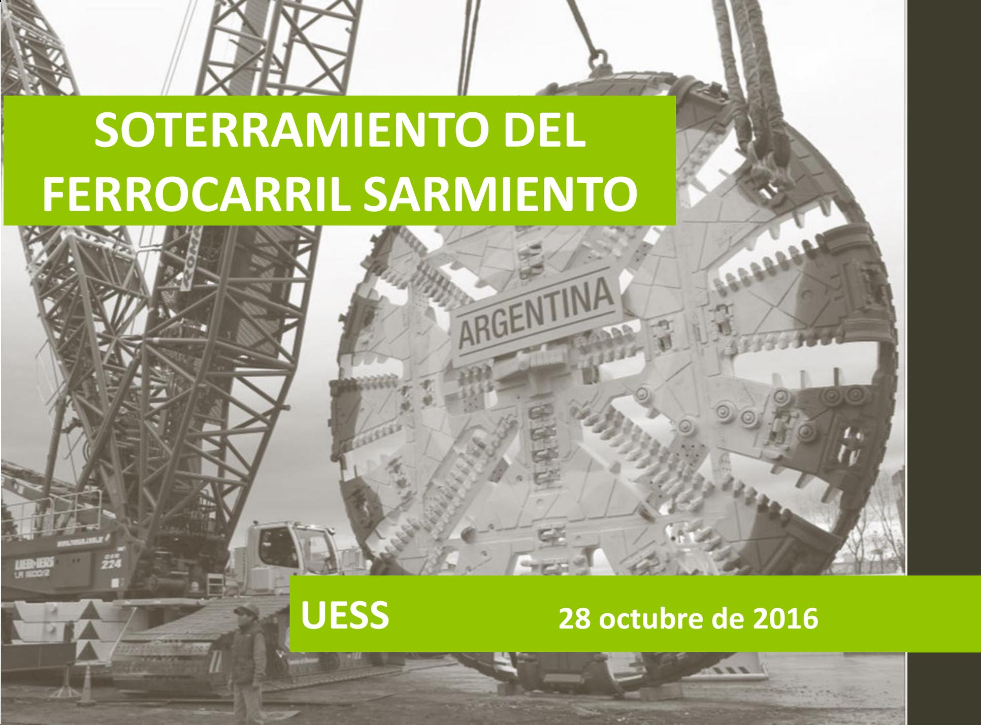
A large circular tunnel boring machine cutterhead is being transported by a Liebherr LR 1800/2 crawler crane. The cutterhead is a complex, circular structure with many cutting tools and is labeled 'ARGENTINA'. The crane is a large, lattice-structured machine with a long boom. The scene is outdoors, likely at a construction site or a port.
